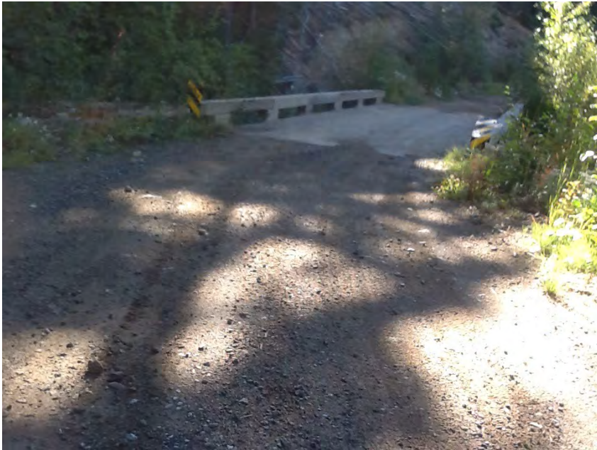
Right approach facing structure
