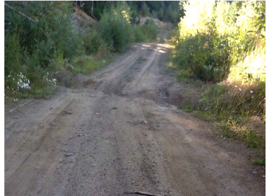
Left approach facing away from structure
