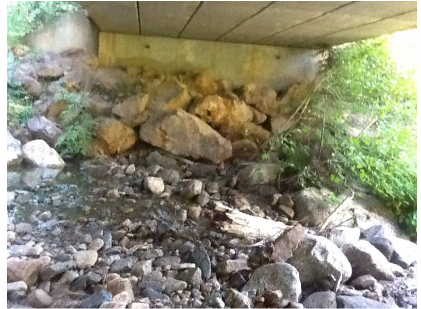
Left Bank Abutment when facing downstream
