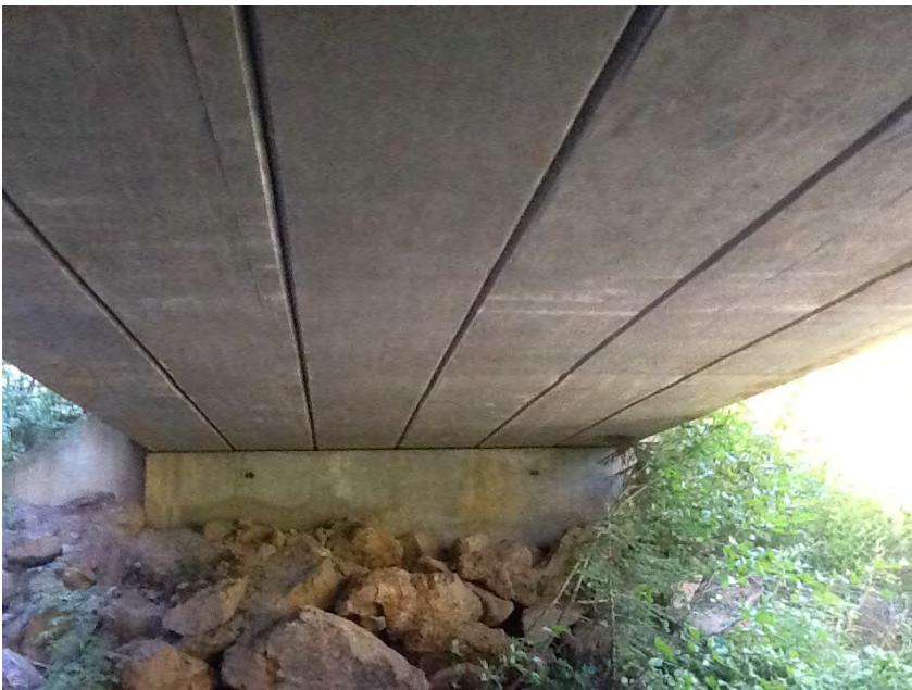
Underside of bridge
