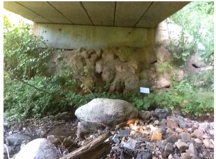
Right Bank Abutment when facing downstream
